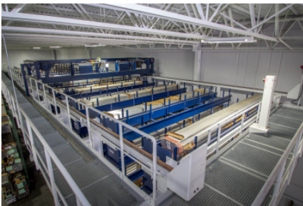
An overhead storage and retrieval unit inserts and retrieves the cassettes in the twelve aisles of the longspan shelving store
