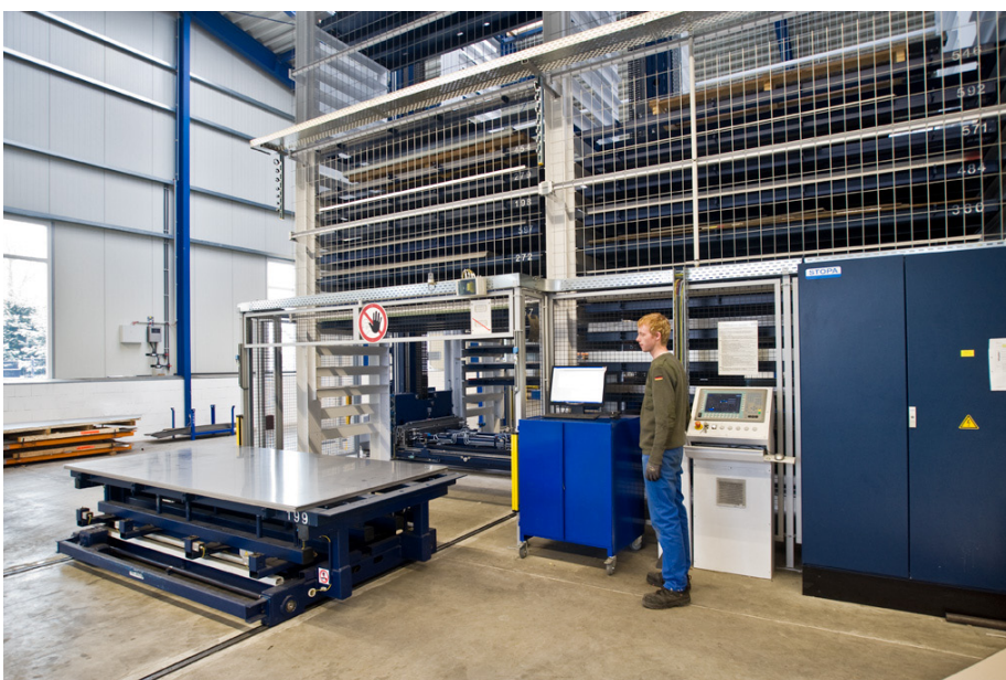
A Schickling employee commands the system to place delivered sheets into storage.
