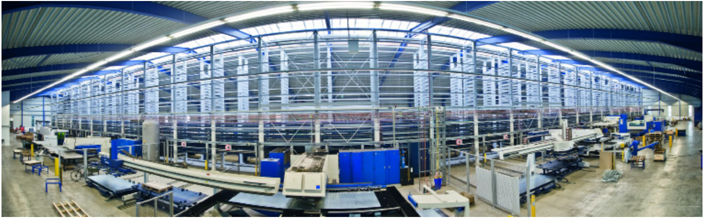
Panoramic view of the STOPA UNIVERSAL storage system at Schickling
