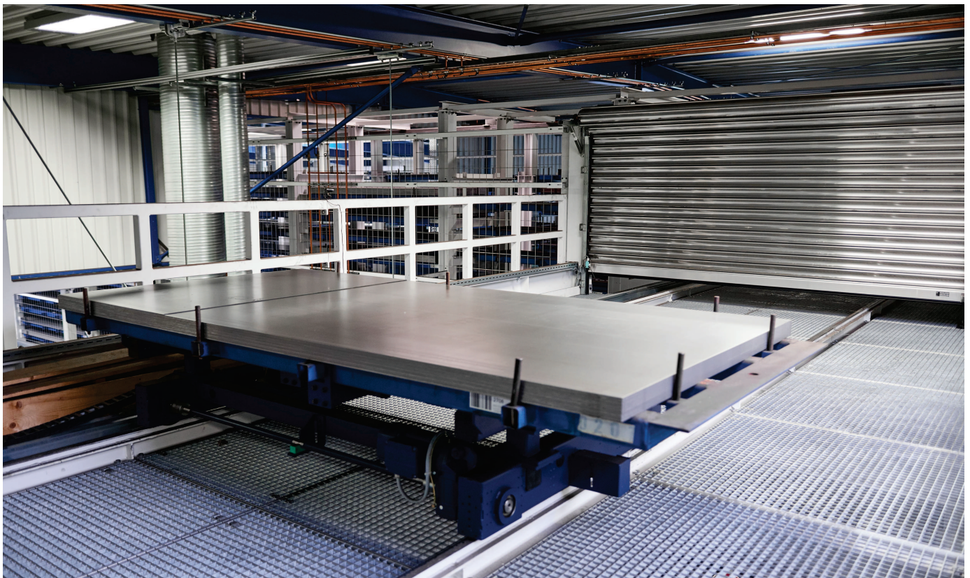
All the laser cutting machines can be supplied with material at any time from either storage system via the bridge-type passageway.
