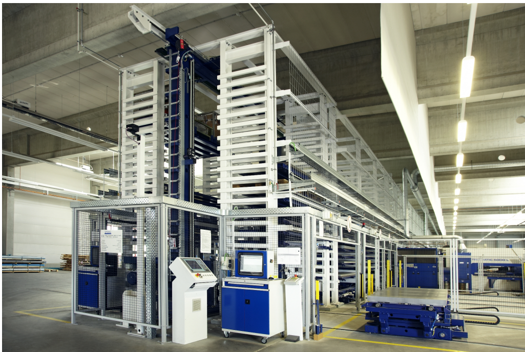
The storage and retrieval unit achieves speeds of up to 150 metres per minute when travelling, 23 when lifting and 20 when pulling or pushing
