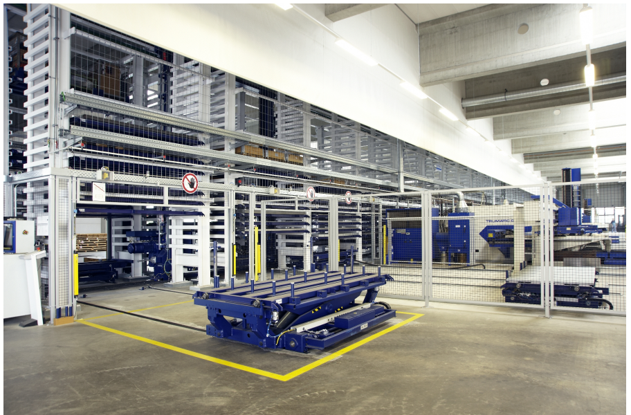
The system is roughly 67.5 metres long and consists of 40 blocks arranged in double rows. It has space for 804 storage locations, not counting the stations
